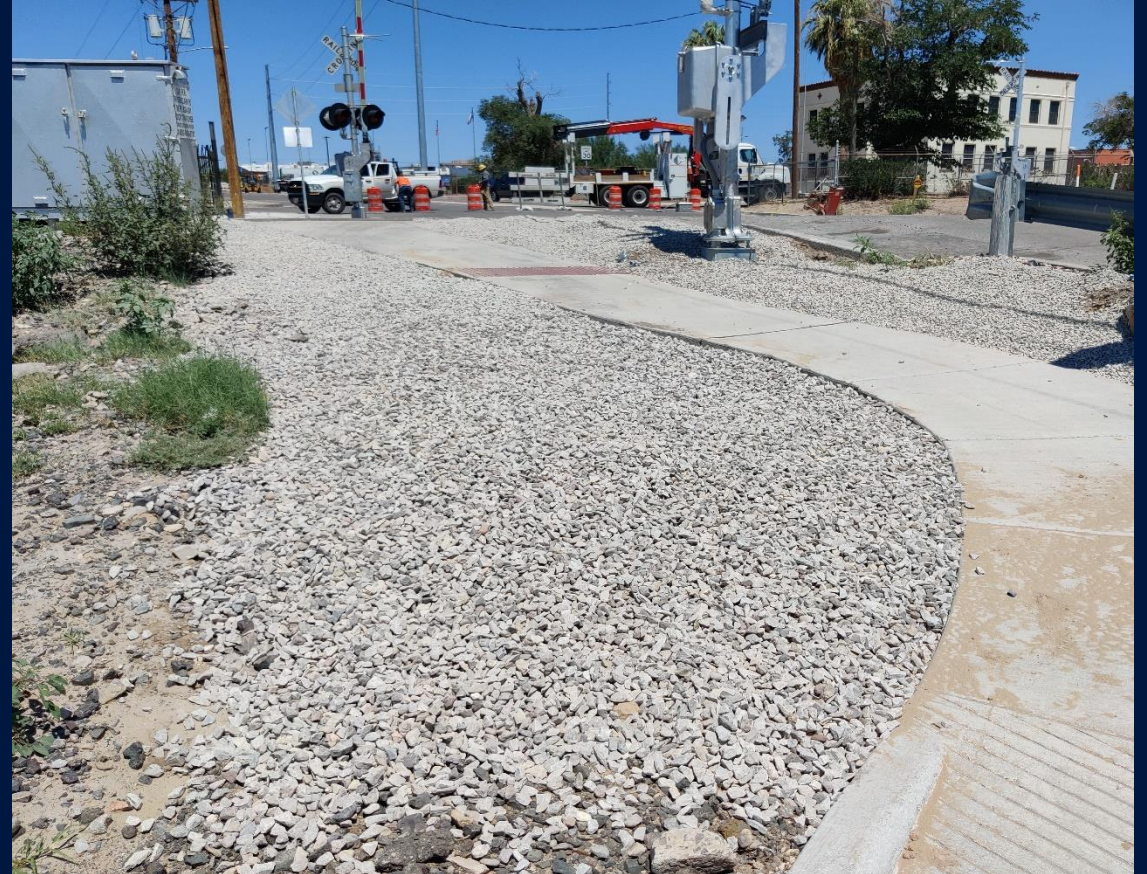
Erosion repair
