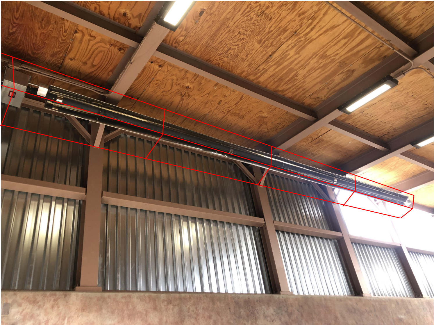
2 x 2 Angle Frame welded to existing structure. Spot weld 2 x 2 wire mesh to angles along length of heater and at ends.
