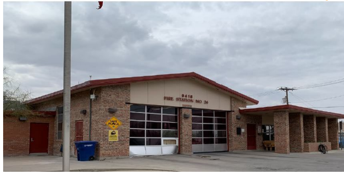
FS 26 Replace Windows and HVAC Upgrade Finishes
