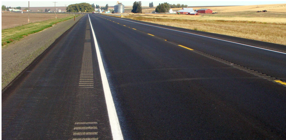
Shoulder rumble strips and center line rumble strips are installed on this roadway.
