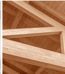
Exposed glulam construction
