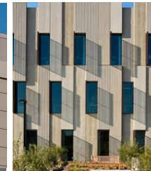
Tilt-up concrete
