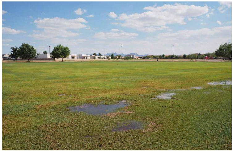
Stormwater ponding at Mary Frances Keisling fields due to oversaturation and clay soils
