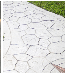
Stamped concrete/Concrete finish
