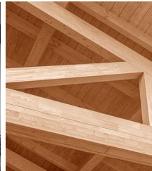
Exposed glulam construction
