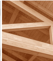
Exposed glulam construction
