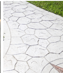
Stamped concrete/Concrete finish
