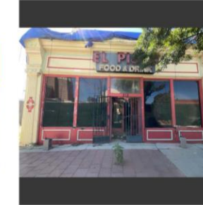
ID No. PA - 14 AKA The Chinese Laundry Address 212 W. Overland Year Built 1901 | Over 50 Owner City of El Paso PID 8360359
