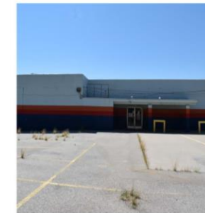
ID No. PA - 19 AKA UK Address 307 S. Santa Fe Year Built 1975 | Less than 50 Owner City of El Paso PID 394786
