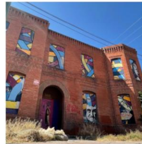
ID No. PA - 01 AKA The Mansion House Address 306 W. Overland Year Built 1904 | Over 50 Owner City of El Paso PID 162938
