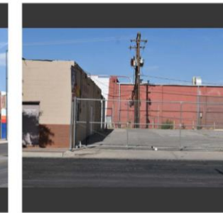
ID No. PA - 21 AKA UK Address 325 S. Santa Fe Year Built Not Listed | Block Shed Owner City of El Paso & Los Paisanos Autobuses PID 47625 & 498575
