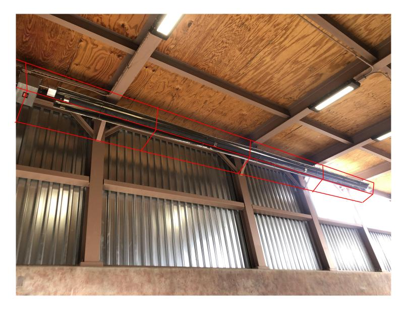
$2 \times 2$  Angle Frame welded to existing structure. Spot weld  $2 \times 2$  wire mesh to angles along length of heater and at ends.
