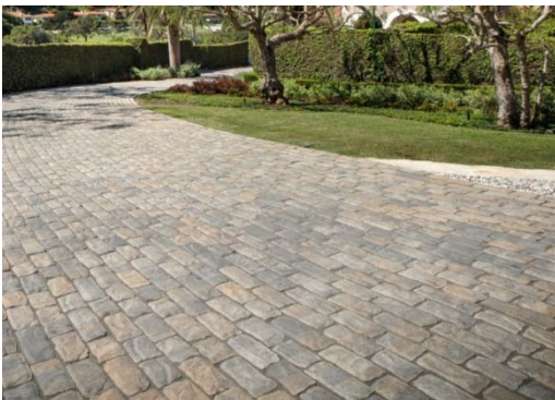
Proposed driveway paving – Concrete paver with cobblestone appearance in color Grigio Gray
