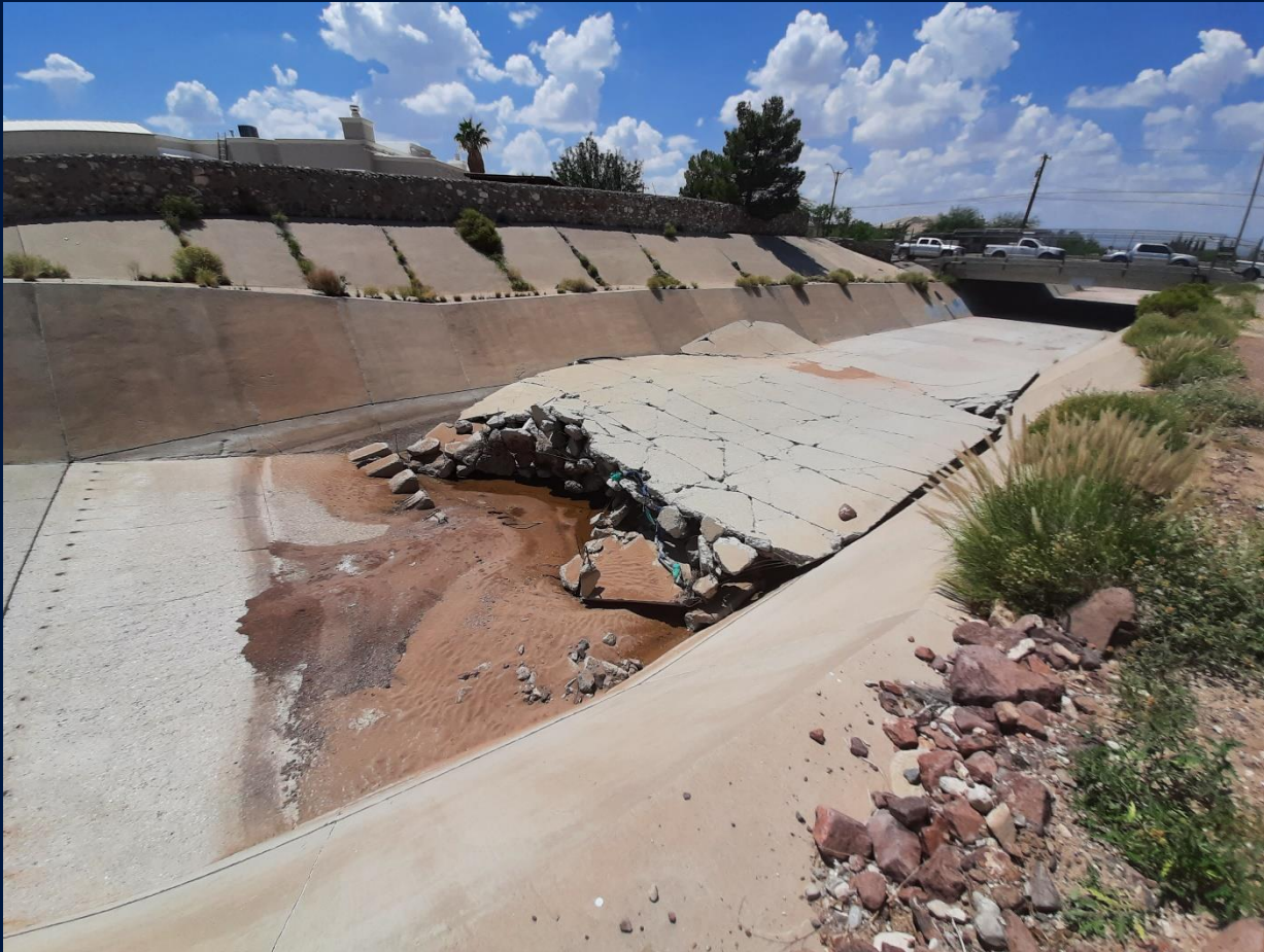
Concrete channel repair
