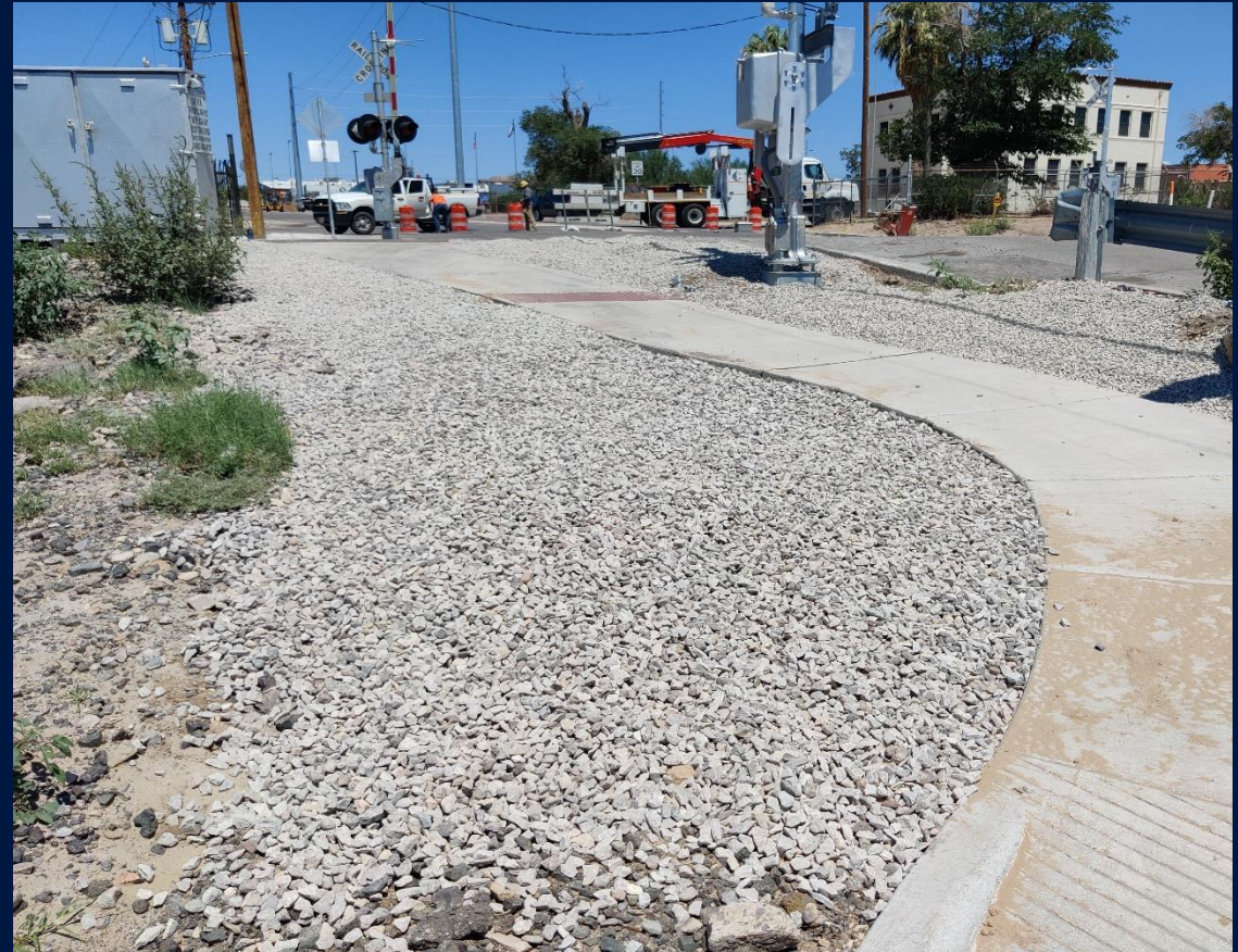
Erosion repair
