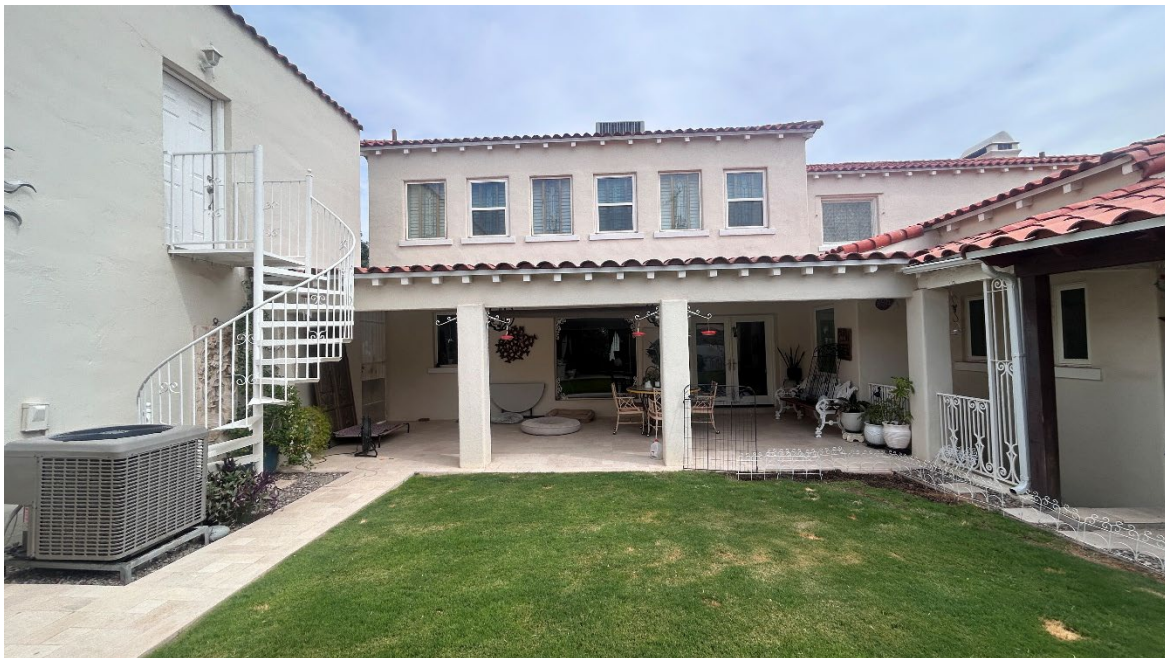
Subject Property (Existing Rear Porch to be Enclosed)
