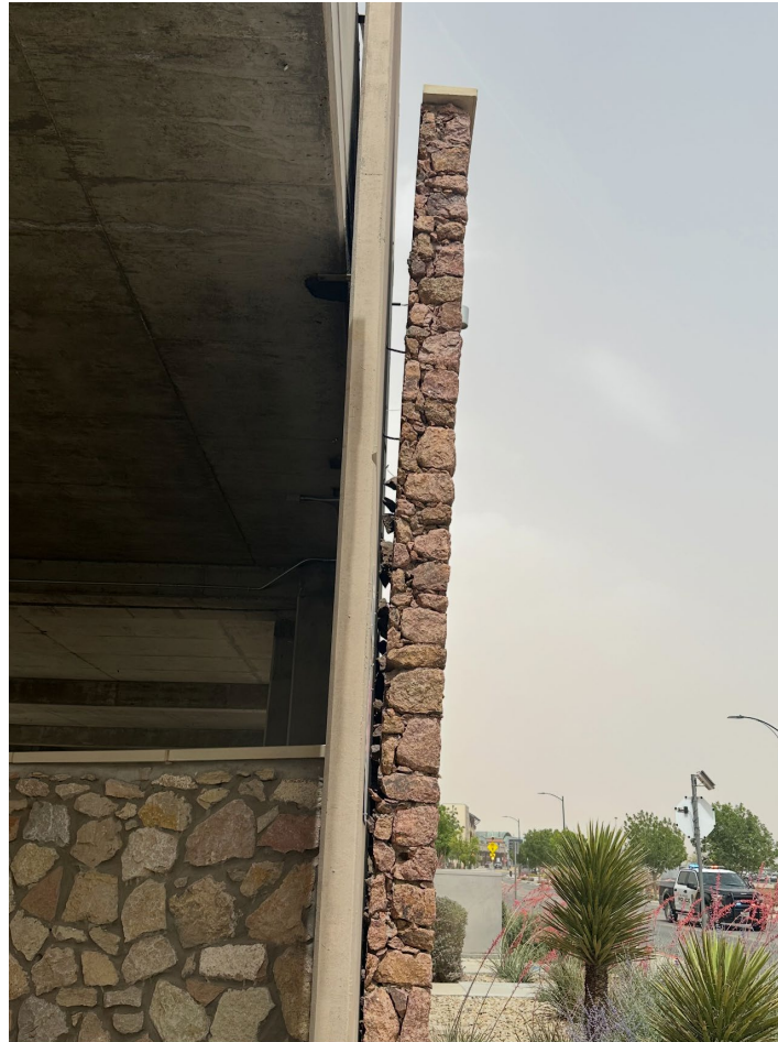
One of three remaining walls showing signs of detaching and collapsing
