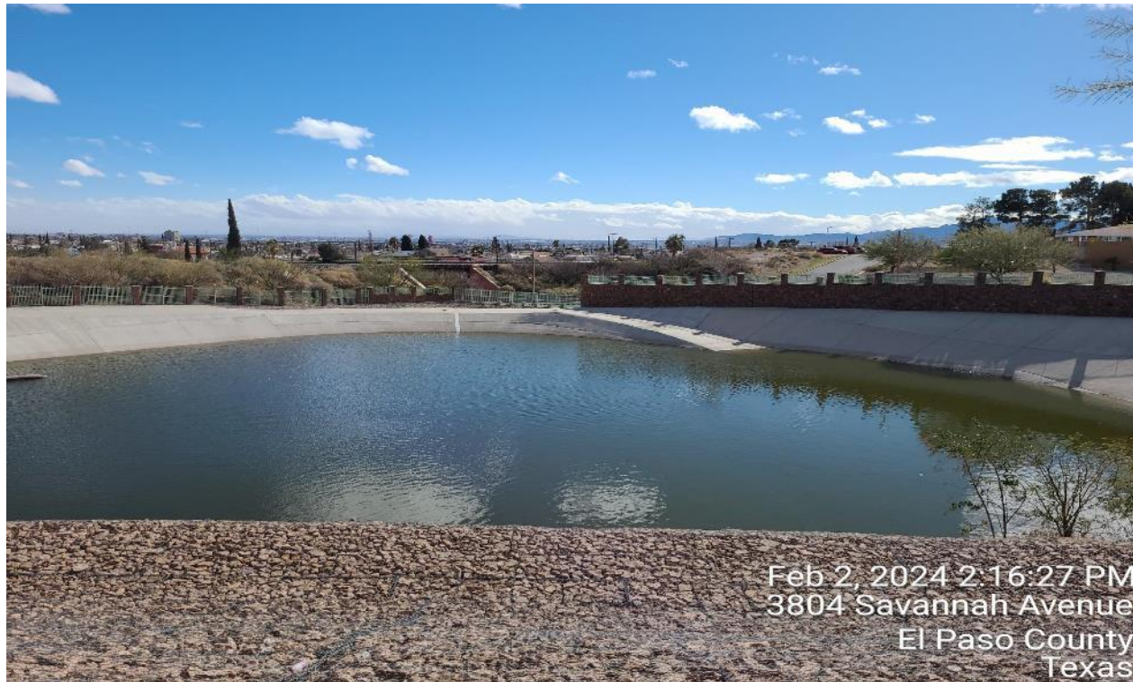
Installation of bleeder line
