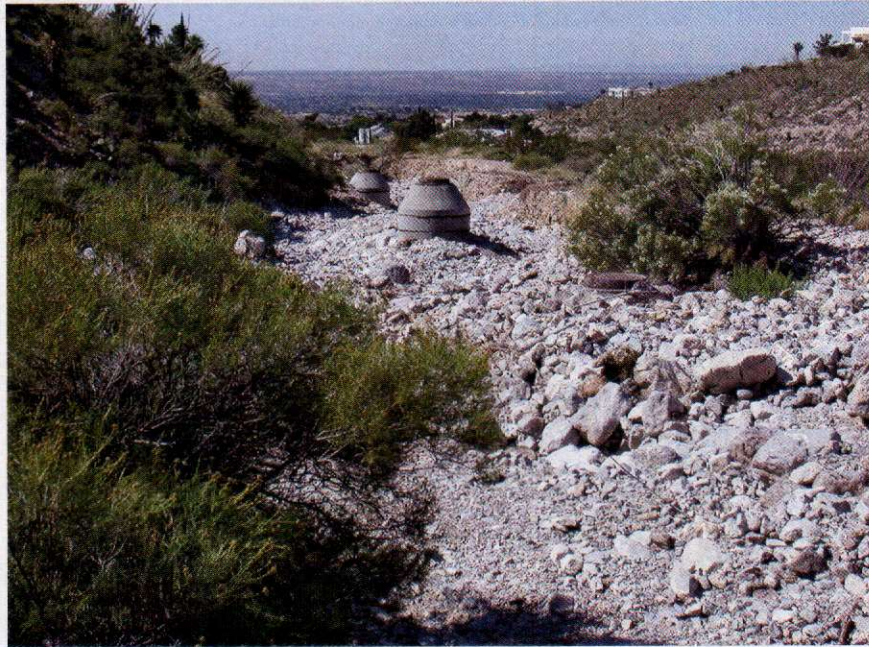
Figure 2. Erosion Around Sewer Line in Thunder Canyon
