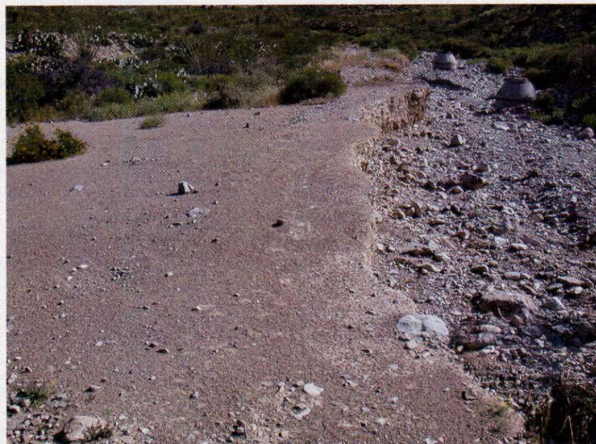
Figure 3. Erosion of Maintenance Road after August 1, 2006 Rainstorm. Maintenance road on left, erosional channel and exposed sewer manholes on right
