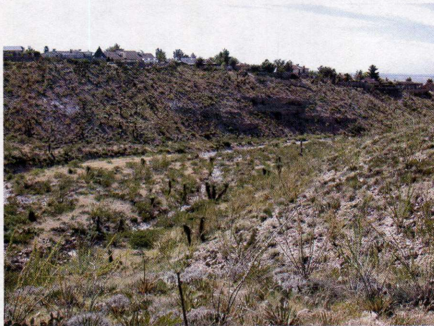
Figure 4. Changed Flow Path in Canyon. Original flow path goes to right side of photograph, new erosional channel on left side of photograph with exposed sewer manhole.
