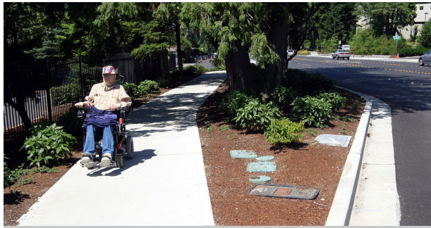
Example of a sidewalk in a residential area.
