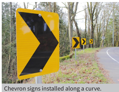
Chevron signs installed along a curve.
