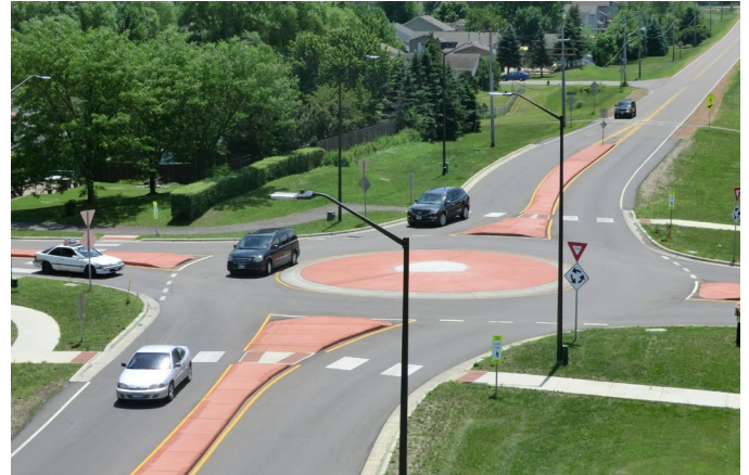
Example of a single-lane roundabout.
