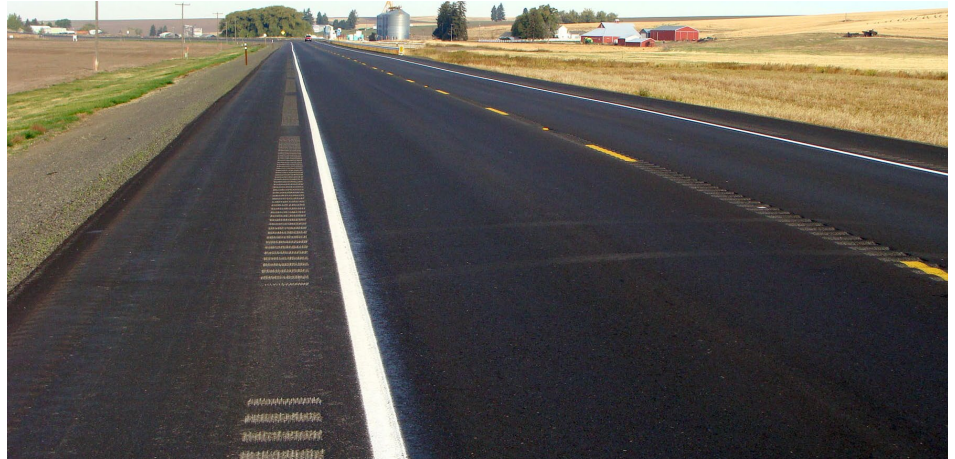
Shoulder rumble strips and center line rumble strips are installed on this roadway.
