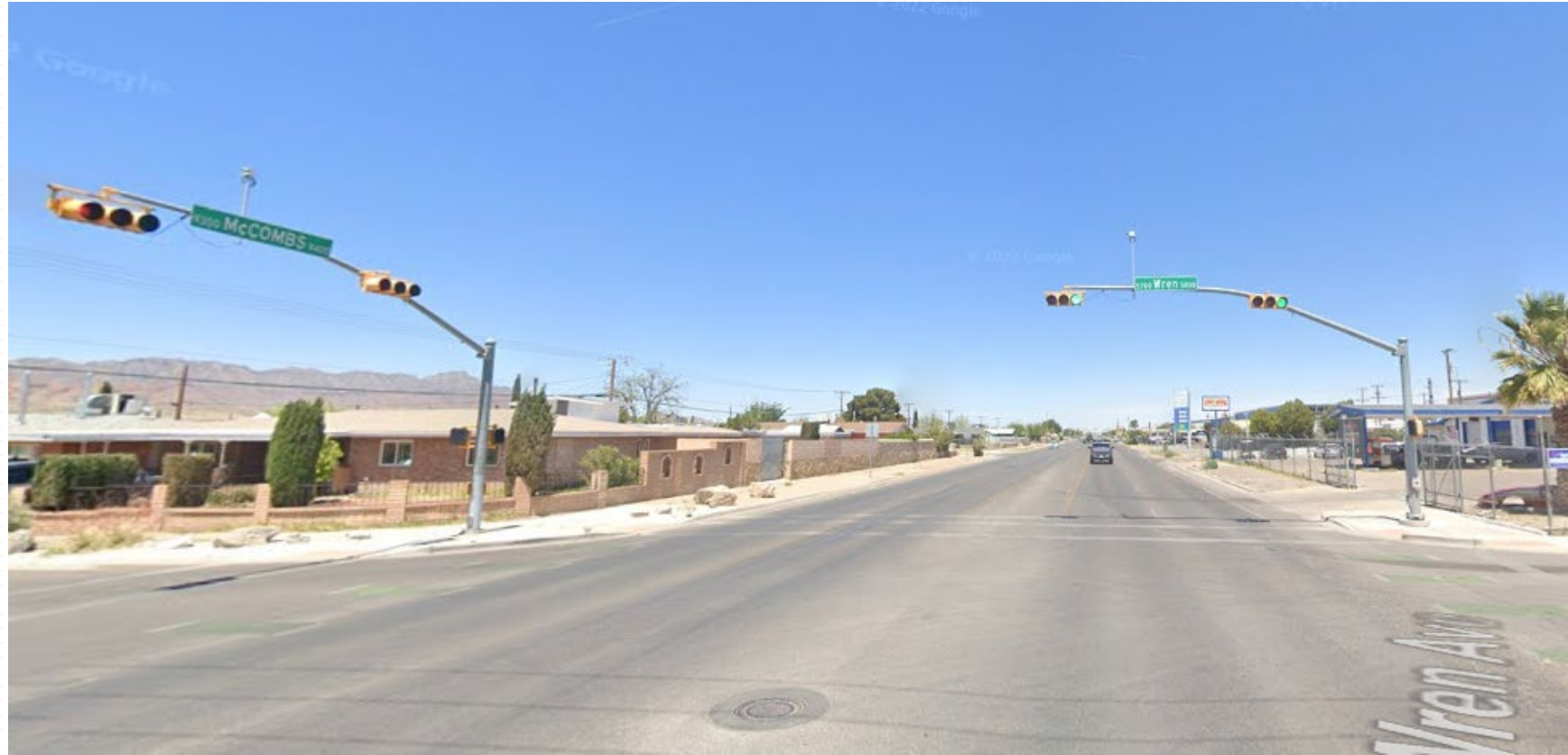
Existing conditions on McCombs St. and Wren Ave.
