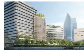
New Goldman Sachs Campus 2 • 800K SF office campus • Broke ground: 2023 • Expected completion: 2027
