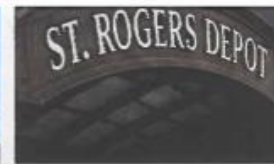
ARCHED FASCIA Curved steel fascia w/ raised lettering. Rivet plate detail adds character and strength.
