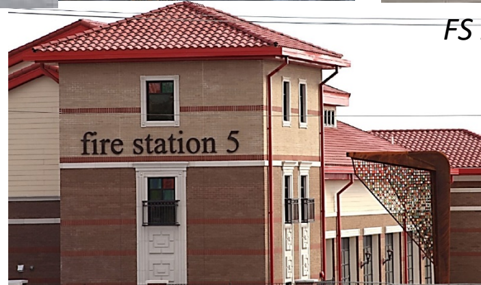
FS 5 and 37 Install Direct Exhaust Capture System
