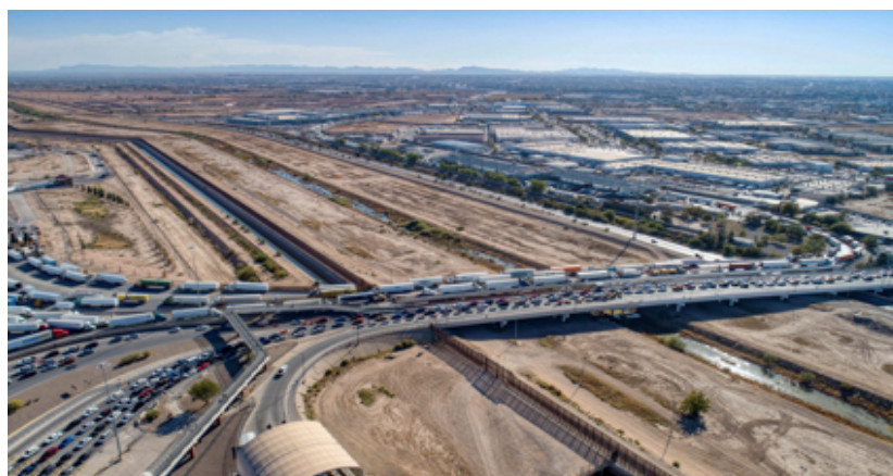
Picture 2. Ysleta / Zaragoza Bridge
