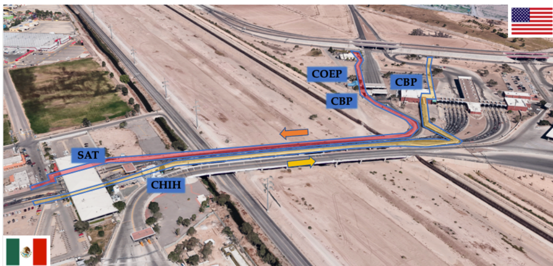
Picture 8: Ysleta/Zaragoza Bridge
