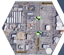
Lee Trevino Median Enhancements_Trawood to Montwood (2020 HSIP Project Awarded Funding, $247,786 construction, 10% City share, for letting of FY 2022)
