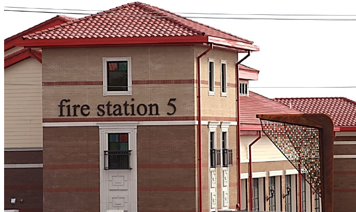
FS 5 and 37 Install Direct Exhaust Capture System
