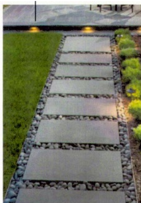
Proposed walkway pavers – 3' x 6' rectangular concrete pavers
