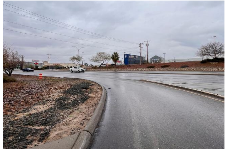
INTERSTATE 10 AT GILES ROAD
