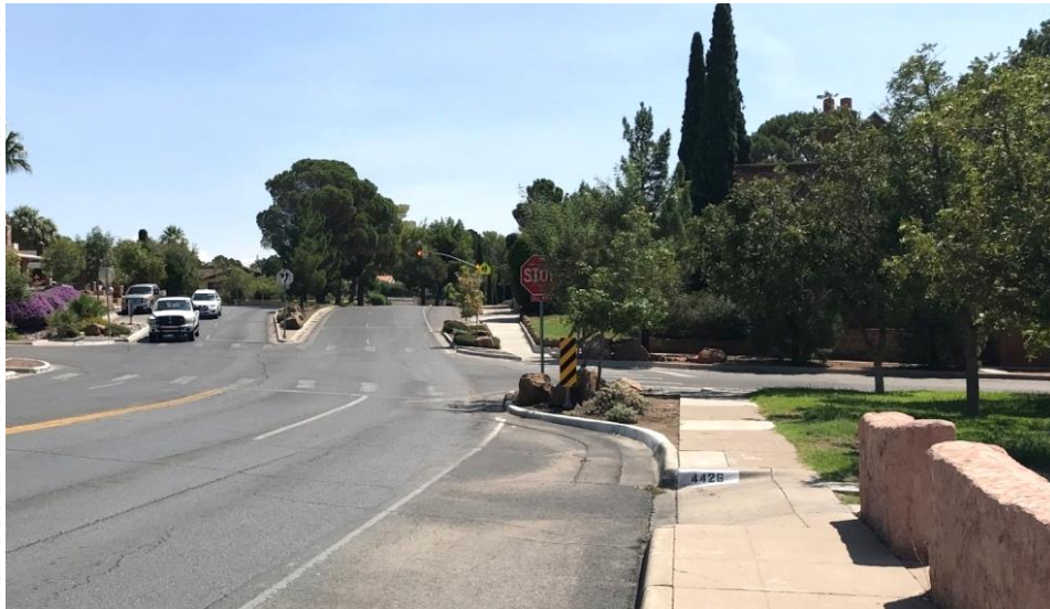
Trowbridge Existing Conditions
