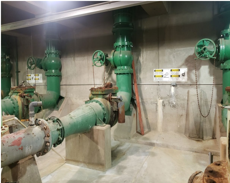
Frontera Lift Station Pump Replacement
