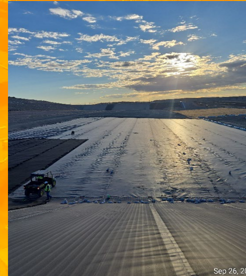
Lining of Landfill Cells
