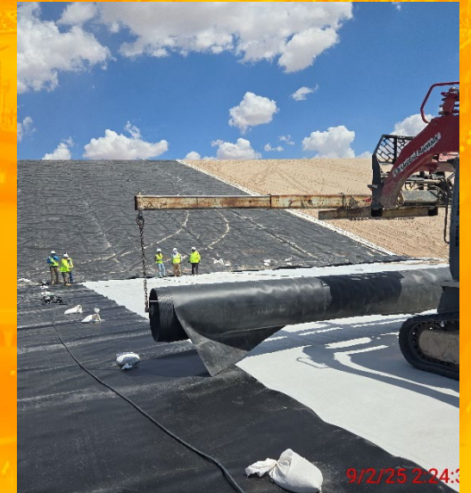
Placement of HDPE
