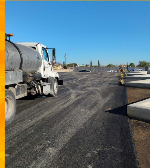
Paving of CCS
