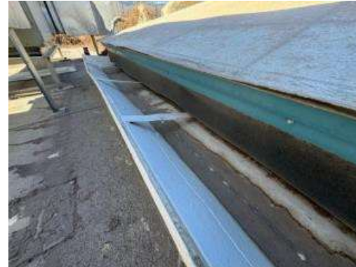
Roof Flashing, Membrane, & Gutter
