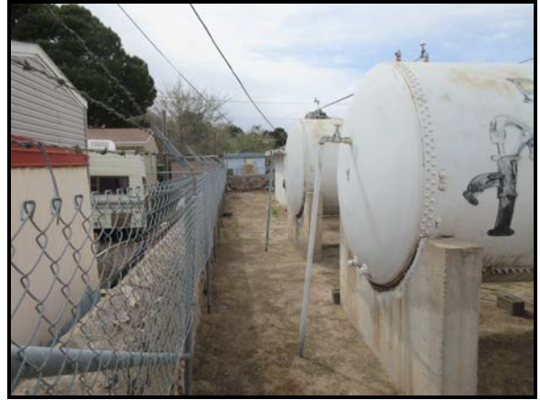
View of the subject site facing west.
