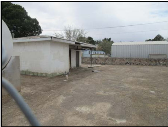
View of the subject site facing west.
