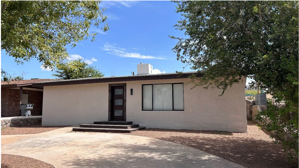
Subject Property (Existing Façade Improvements approved on August 14, 2024)
