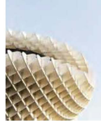
Exposed glulam construction
