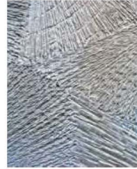
Stamped concrete/ Concrete finishing
