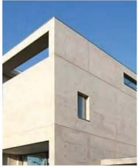
Cast in place concrete
