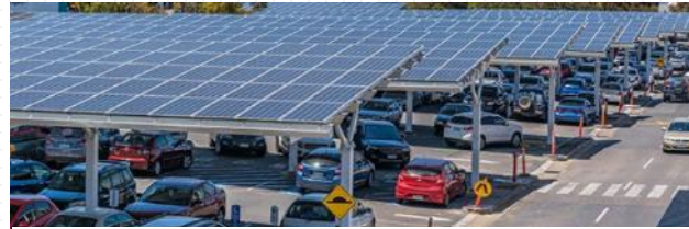
Solar Parking (Microgrid)
