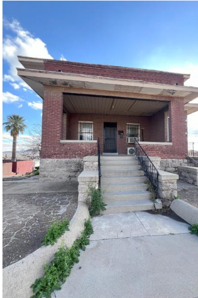
North - Main Bldg Entrance
