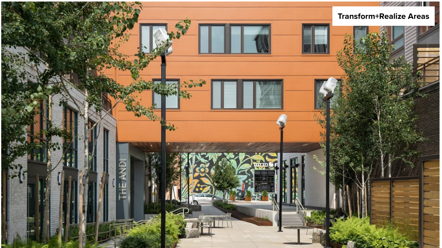
The fiber cement color, linear pattern, and window frame composition add visual interest to the building architecture.
