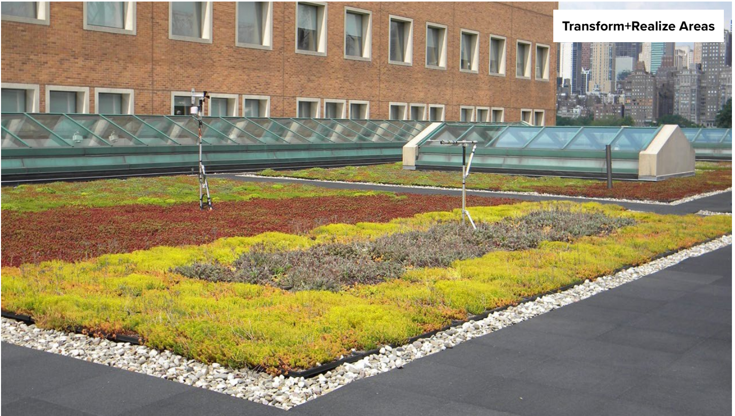
Horizontal roofs are recommended to include green infrastructure for stormwater.
