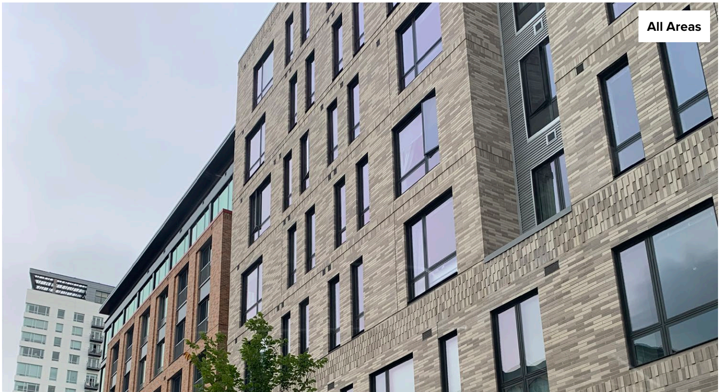
Brick soldier courses, stepping in and out, variation in the masonry itself, and deep recesses and insets add richness to the façade.
