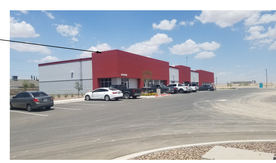
6 A.I.O. EXISTING BUILDING 'B' N.T.S.
