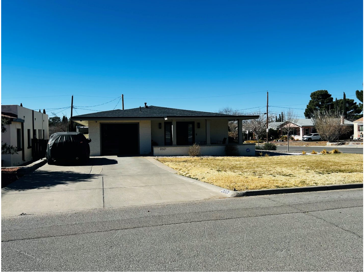
Subject Property | Front view facing Ochoa Street
